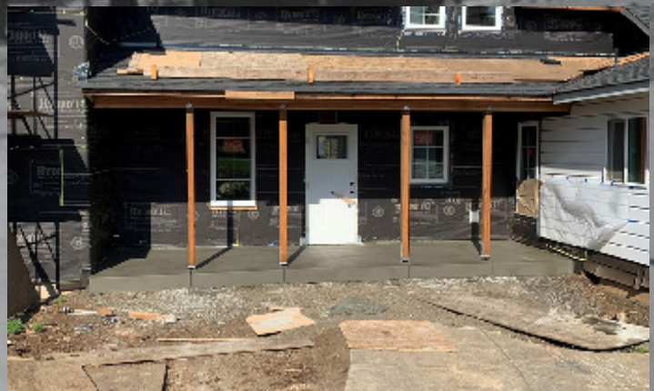
The same porch after adding footings and a foundation. The porch was sagging and also needed to be rebuilt.
