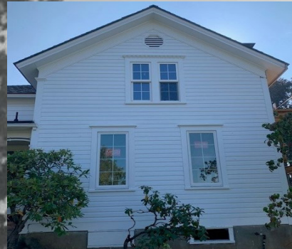
Original House (Note two small windows in basement)
